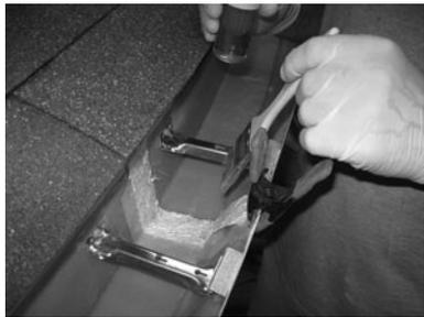
3. Pour about 1/4 of the resin hardener mixture on to the lap joint and spread with brush along front and back. Apply a strip of fiberglass on to the lap joint, making sure half is on the lap joint and half is on the adjoining piece. Pour the remaining amount of resin on to the lap joint and spread evenly with the brush, making sure to dab the top, the front, and the back bead. Spread the excess resin along the inside of the gutter.
